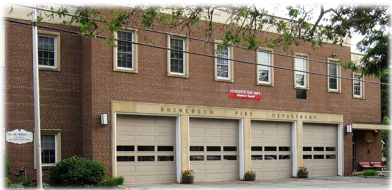
Rhinebeck Village Hall and Fire Department, East Market Street. Photo by Michael Forlenza.
